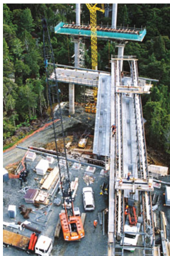
A beam is launched for the first span of the eco-viaduct.
