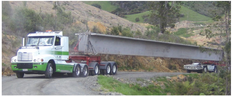
A bridge beam makes its way to the launching site.
