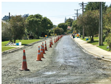
Otanerua Road during the upgrade works in November this year.
