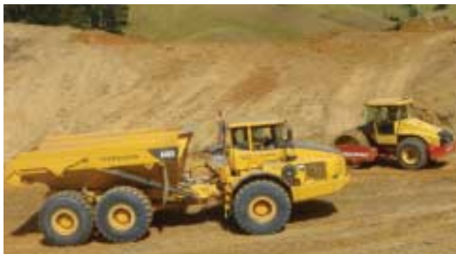
The graduate earthworks operators are now at work on ALPURT B2
