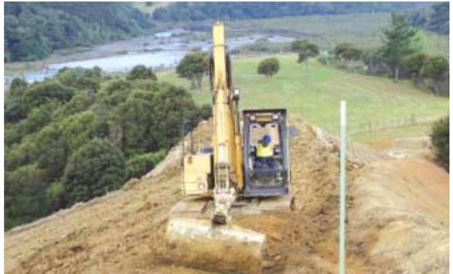
Haul road under construction in Section B
